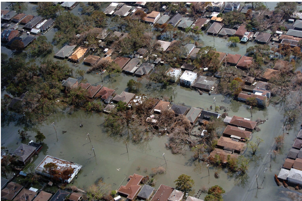
Figure 1.1 Flood Damage After Hurricane Katrina, 2005
